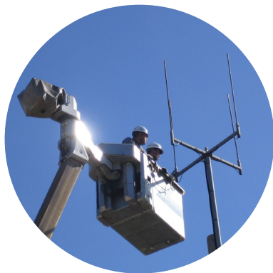
Installation of PHS antenna
