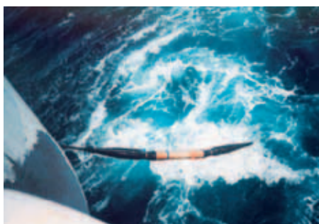
Laying a submarine cable repeater
