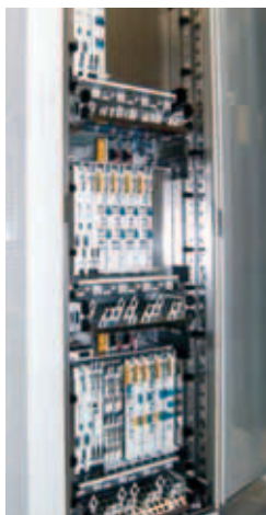
Installation of main submarine terminal equipment
