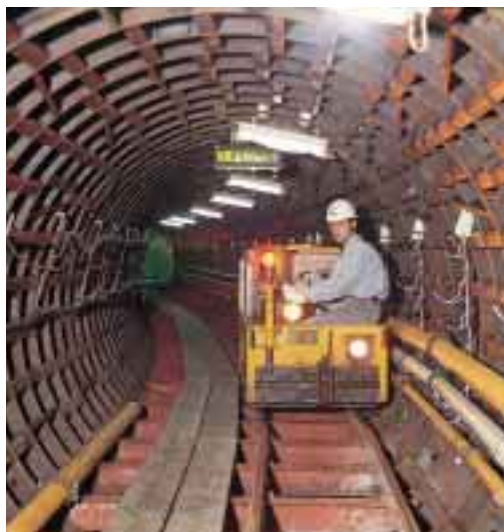
A cable vault ready to receive telecommunications cables.
