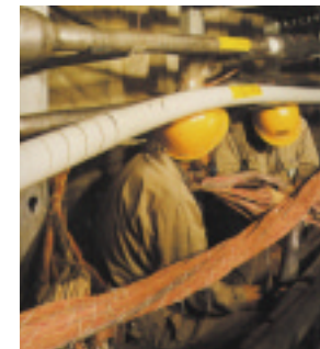
Cable conversion project (1978)
