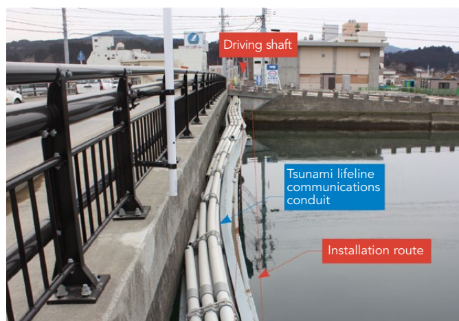
Installing communications cable under the riverbed at Shiomi Bridge (A new underground conduit was drilled at a depth of 11 m, and a telecommunications cable was laid across the river under the riverbed.) The driving shaft for initiating the Acemole method was dug on the far side of the river.
