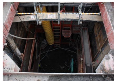
Driving shaft for initiating the Acemole method
