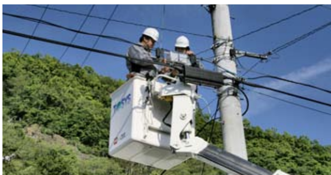
Installation of fiber optic cable
