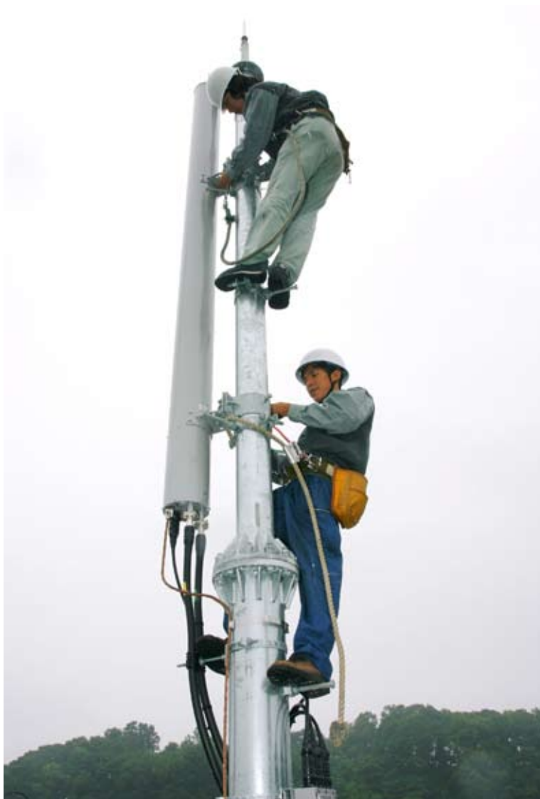
Installation of mobile phone base station antennas
