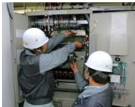
Installation of power supply equipment for mobile phone base stations
