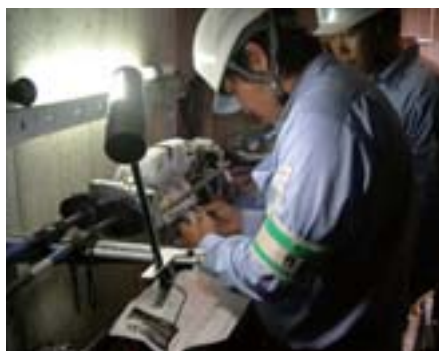
Underground installation of fiber optic cable
