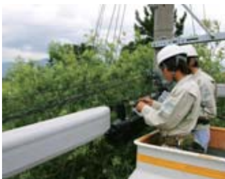
Communications line construction (laying of optical cables for B FLET'S )
