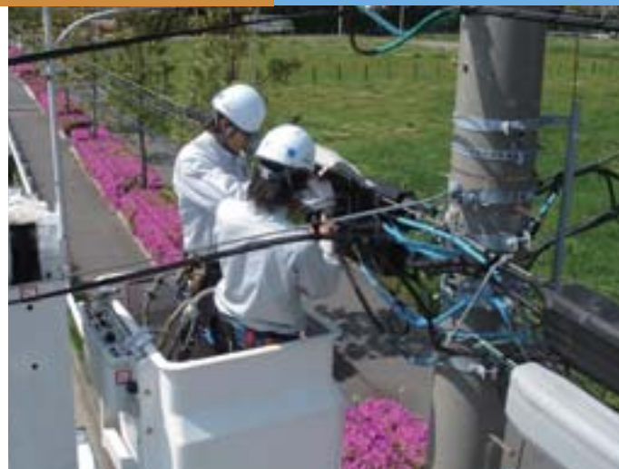
Communication construction work in progress (installation of fiber optic cables)
